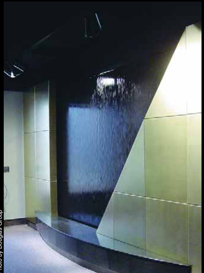
Figure 7: Waterwalls are a lighting challenge best met through use of non-submersible lights – as in this case, where lighting from above creates strong yet subtle impressions by calling attention to tiny ripples and variations in the flow down the wall.
