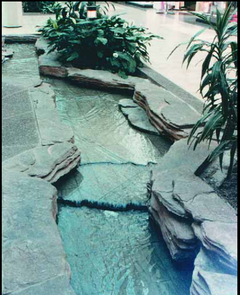
Figure 2: When it comes to illumination, sloped water spillways are among the most challenging of all water effects. Fiberoptic lighting has definitely simplified the process because of its compact nature and the fact that it doesn't heat up the way conventional lighting fixtures do.
