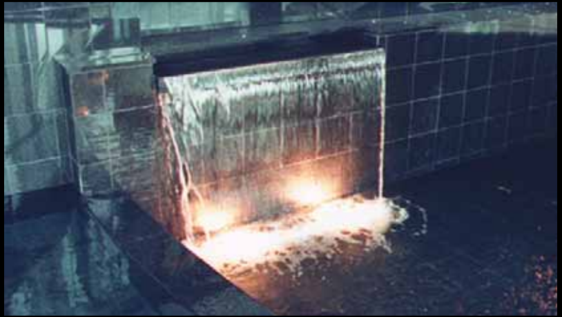
Figure 1: Many waterfalls are designed with water drops of six feet or less. In these cases, you can position light fixtures in front or behind the water to good effect – so long as you keep them away from the foamy water.
